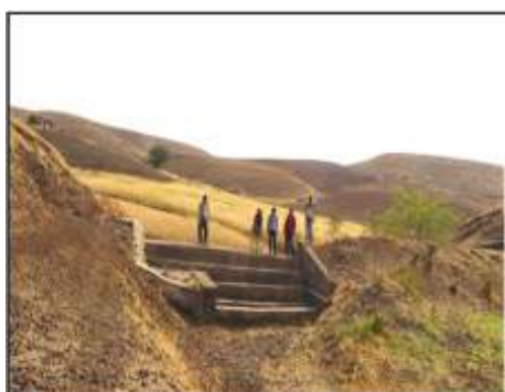
Fig. 3.7.3. Low cost rainwater harvesting-cum-groundwater recharging structure at Doongri para
