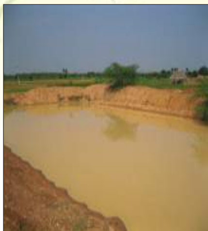
Construction of rainwater harvesting structure
