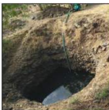
Fig. 3.7.4. Post-monsoon water table in well near low cost rainwater harvesting-cum-groundwater recharging structure at Doongri para
