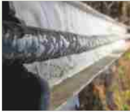
Placement of oozing pipe on PVC trough (trough length-1 m)
