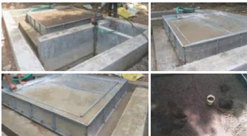
Plate 3.1.4. View of the online screen-gravel filter
