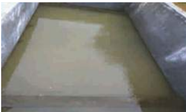
Plate. 3.1.2. Functioning filter during runoff event
