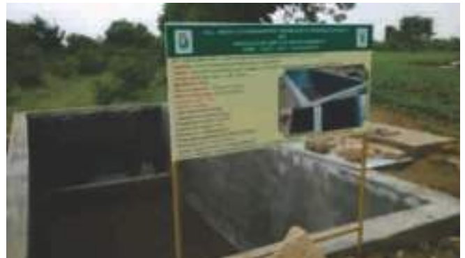
Plate 3.1.1. Execution of connector well system
