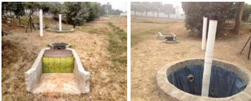
Plate 4.4.1. Testing composte filter in field condition
