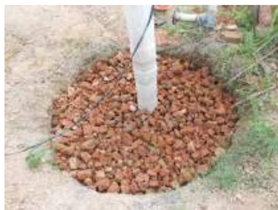
Fourth layer of brick flakes
