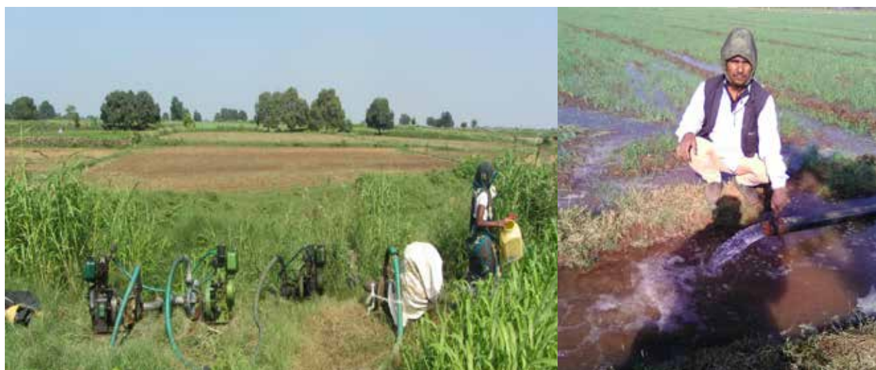
Plate K3. Water carrying through pipe lines from local River for irrigation
