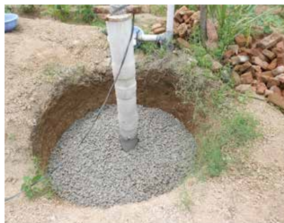
Second layer of angular gravels
