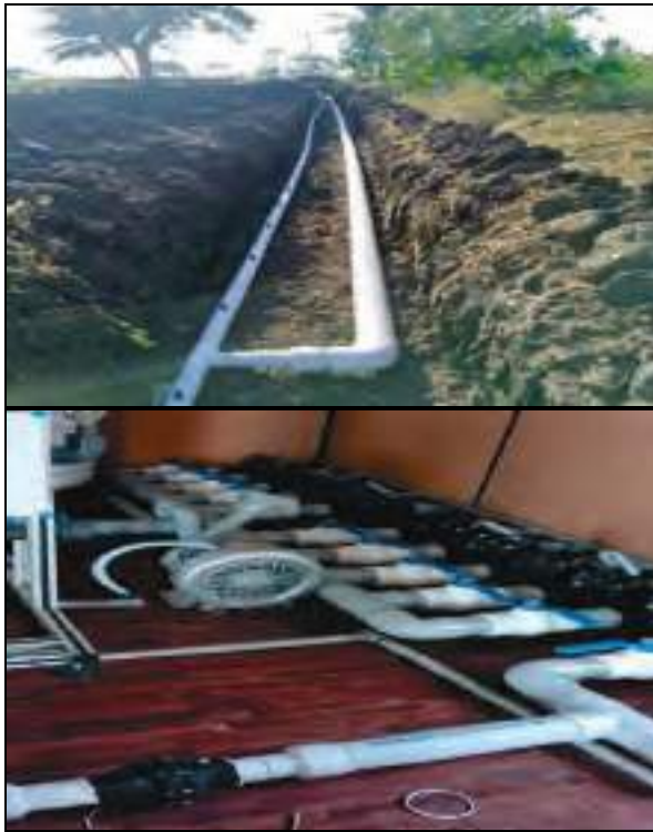
Installation of drip automation unit
