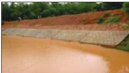
Earthen check dam with stone patching : a case study in Bahasuni watershed, Dhenkanal
