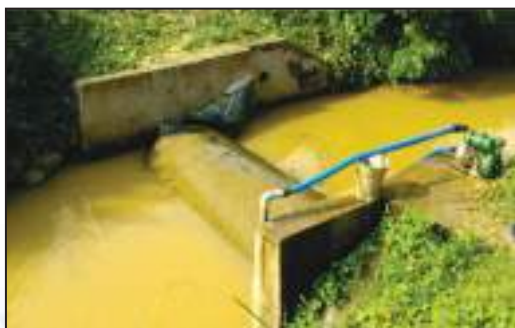
Rubber dams installed in the farmers' field
