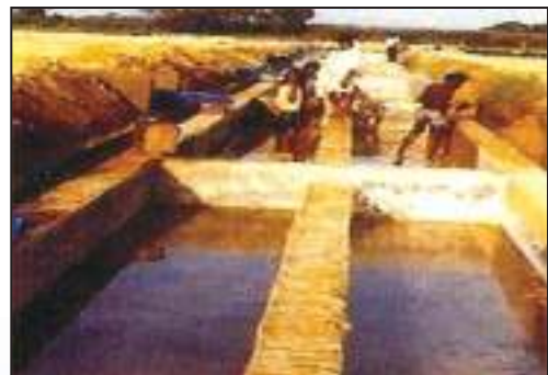
Increased dyke height for in-situ rainwater conservation
