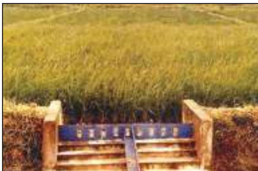
Increased dyke height for in-situ rainwater conservation
