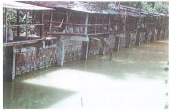
Fig. 10. Renovated poultry sheds after super cyclone
