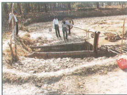
Photo 3 : Construction of open dugwell in progress
