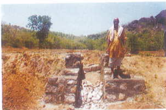
Plate 5. Land modification with stone masonry spillway.
