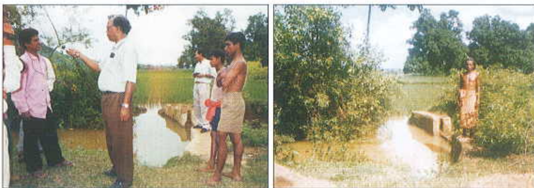
Plate 3. Masonry check dam at Kurumbankatara ashram
