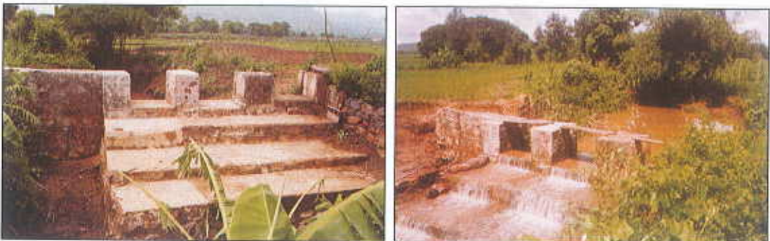
Plate 8. Diversion weir on Nagarina.
