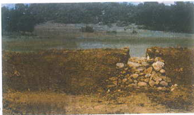
Plate 4. Contour bunding with spillway.
