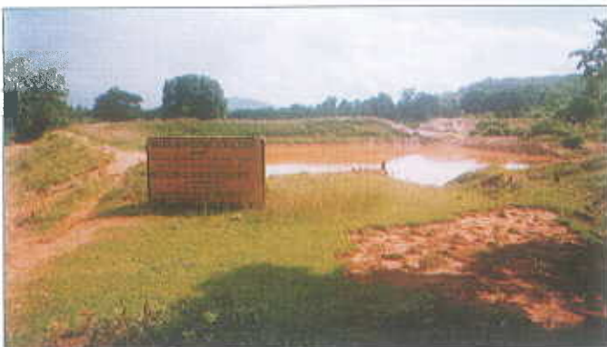
Plate 2. Water Harvesting tank near Paikbanakatara village
