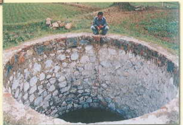
Water level measurement in open dugwell in the watershed
