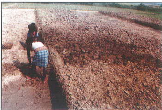
Construction of alternate raised and sunken beds
