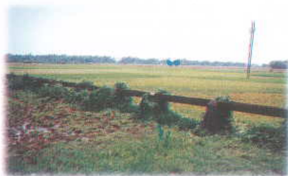
Pipeline to take water from lift point to outlet near the crop field
