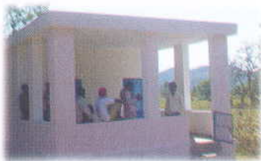
Pani Panchayat building
