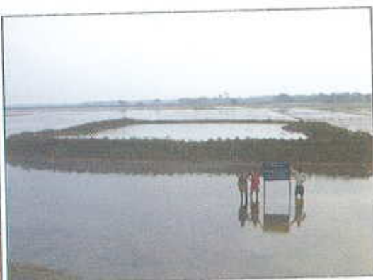
Photo - 6 (d) : View of pond after full recede of accumulated water. The pond is full of water.
