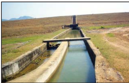
Plate 1 : Koska MIP reservoir embankment and main canal system
