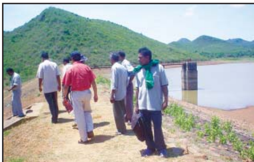
Plate 3 : Reservoir and embankment of Devijhar MIP.
