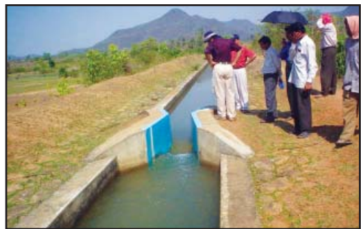
Plate 2 : Flow measuring flume in the Koska MIP canal system
