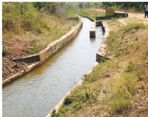
Plate 2. Minor canal (right side) off-taking from the main canal of Devijhar MIP.
