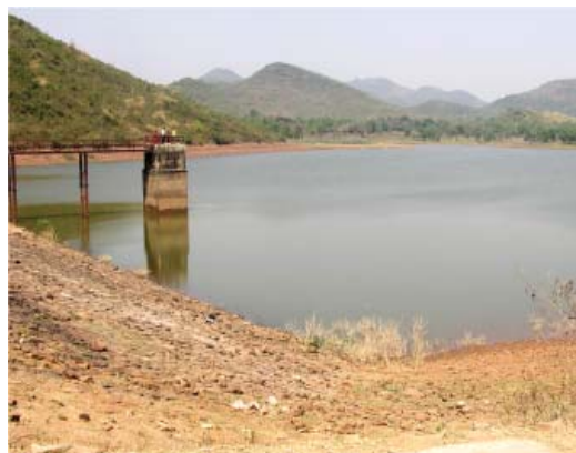
Plate 1. A view of the reservoir of Devijhar Minor Irrigation Project
